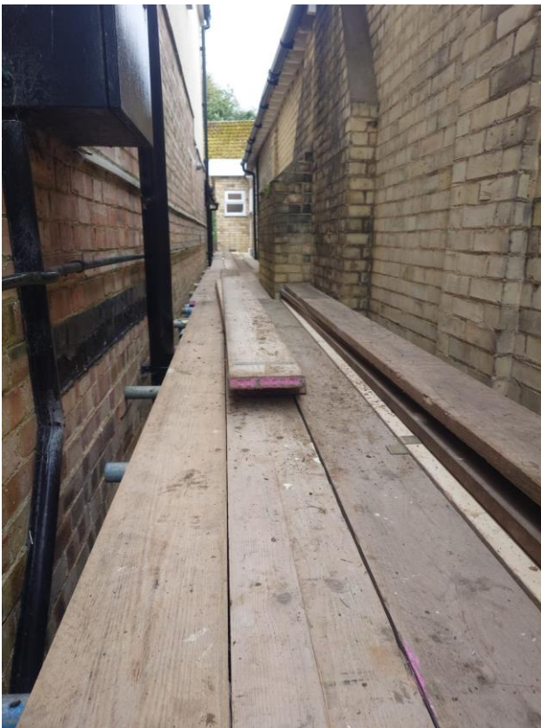
Scaffold access run for waste disposal/materials delivery.
