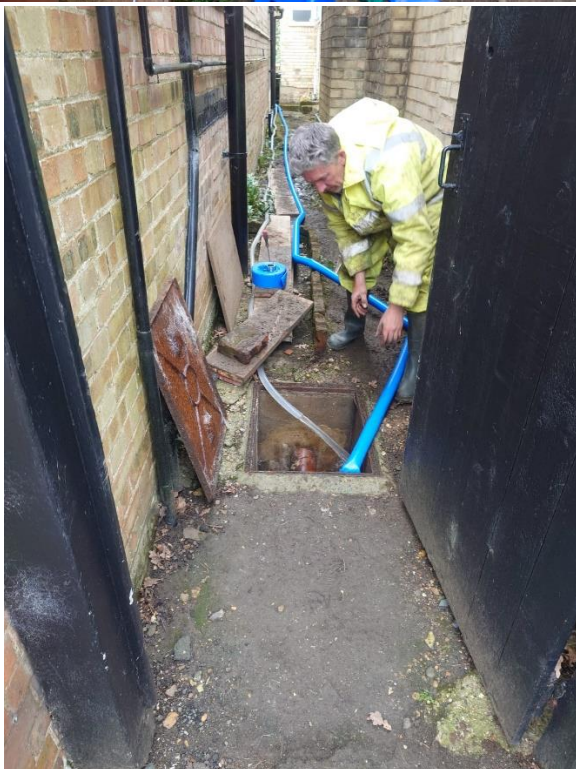
Setting up pumps prior to scaffold erection
