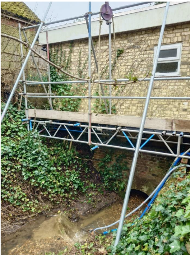
Scaffold erected over culvert.
