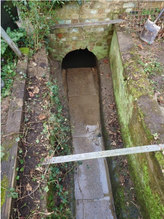
Cover removed showing clear culvert base prior to forming working space.
