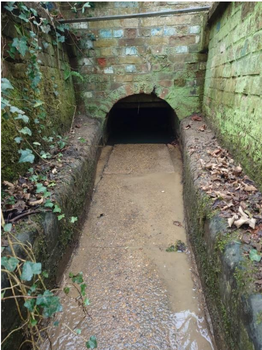
After cleaning out sediment, prior to breaking out working space.
