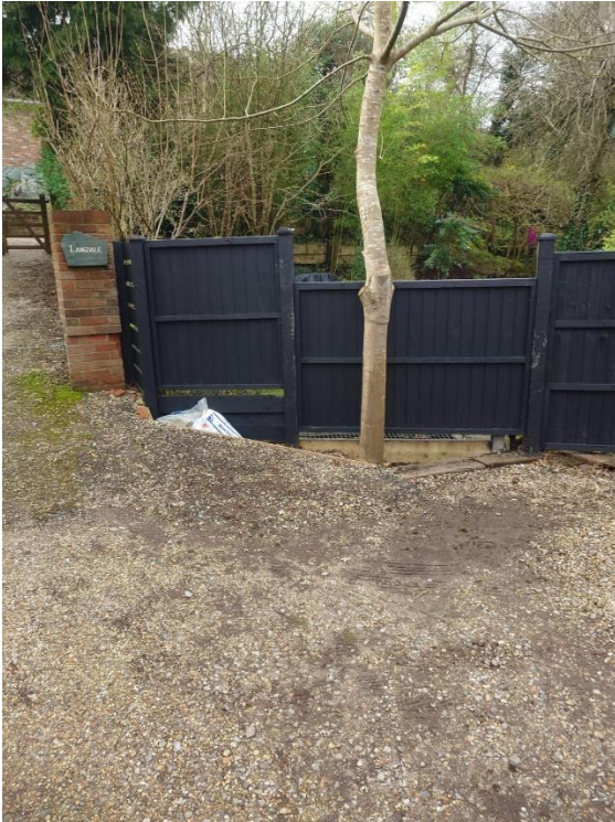
Access via lowered fence panel – remove and replace daily.
