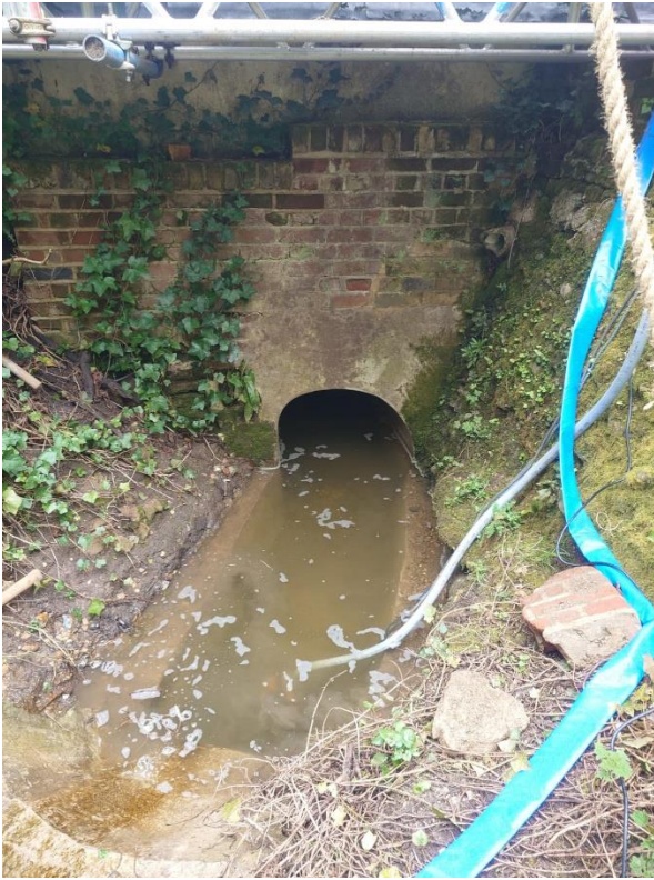
Sediment removed from catch pit and into culvert.
