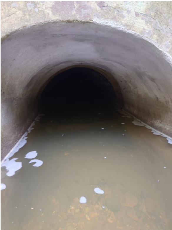
View into culvert from upstream end following sediment removal.
