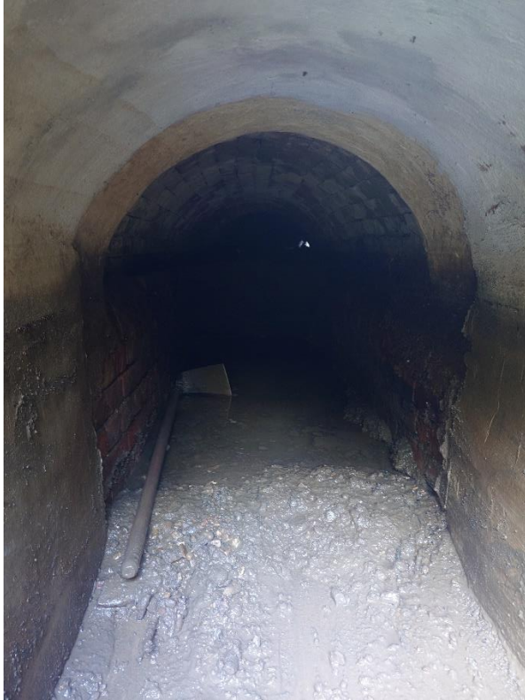
View from upstream entrance to culvert.
