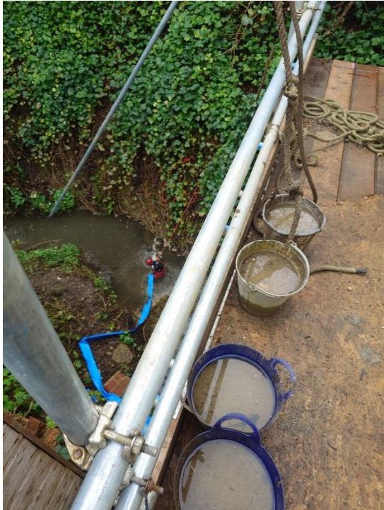
Scaffold access way with sediment removal in progress.
