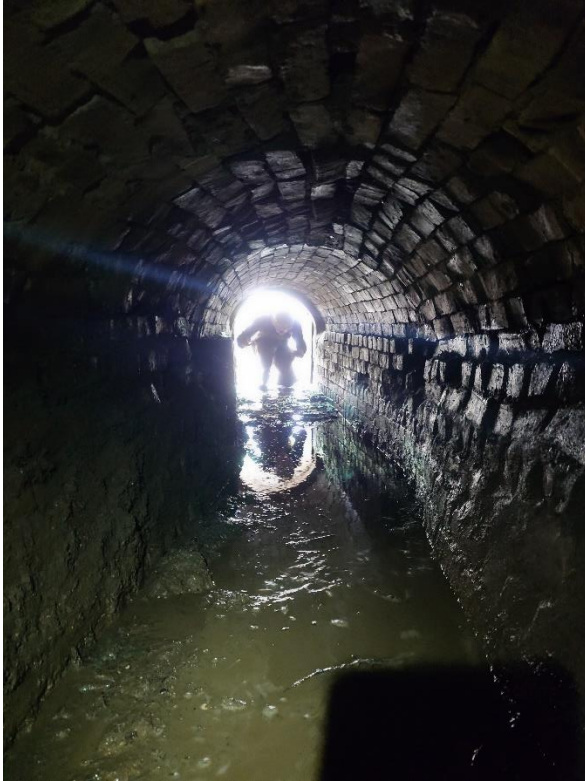
View upstream following sediment removal.
