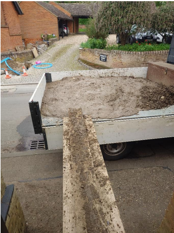
Material loaded for removal from site.
