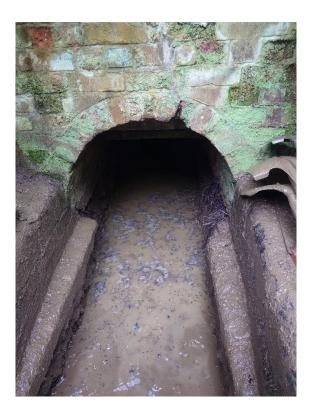
View at culvert invert level showing daylight at upstream end.
