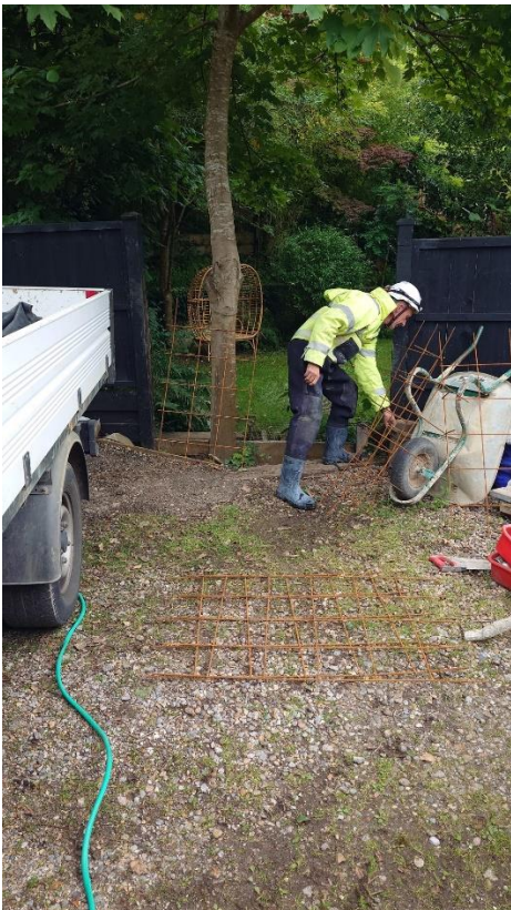
Steel reinforcement preparation
