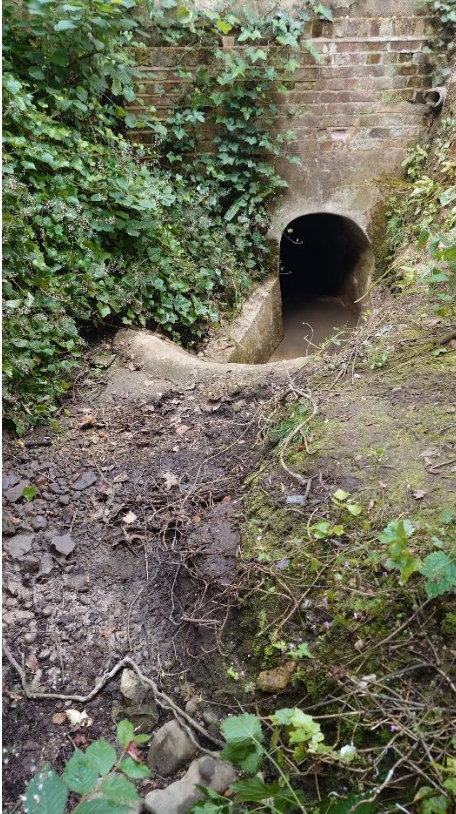
View from further upstream and side passage clear.
