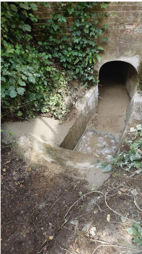
Concrete repairs completed to upstream.
