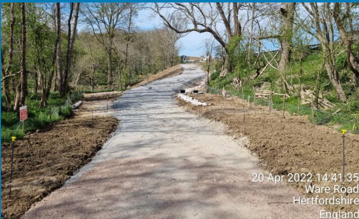
Cycle track construction progress
