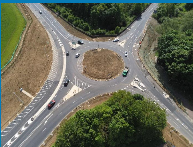
A602 roundabout at completion
