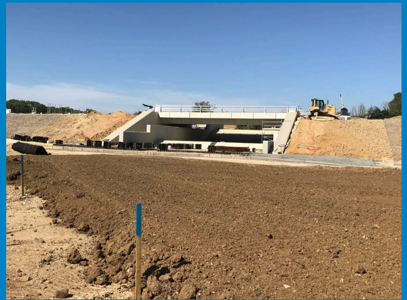
Albury Tributary reservoir spillway
