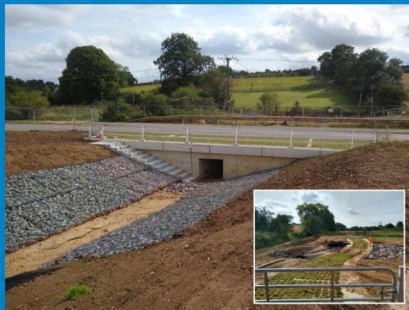
Lloyd Taylor Drain. Laying of Grasscrete inset
