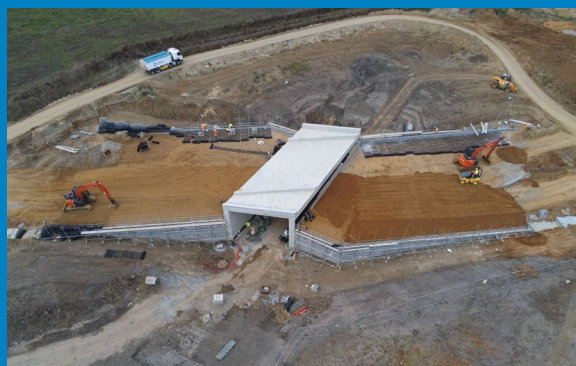
Hadham Park Underpass from above
