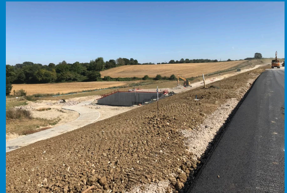
The northern side of the River Ash embankment
