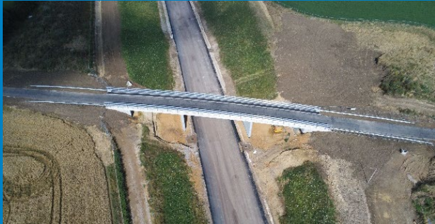
Mill Mound Bridge
